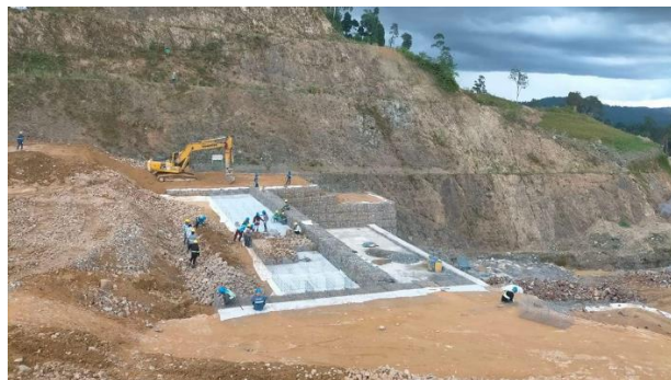
Mattress installation RL450 on April 26, 2022.
