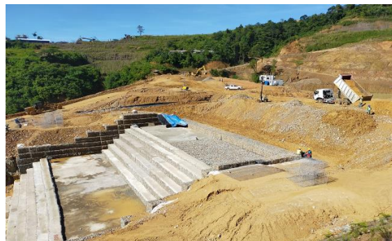
Gabion installation RL451 on May 5, 2022.
