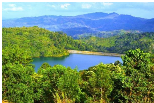
Canatuan Tailings Storage Facility – June 2021
