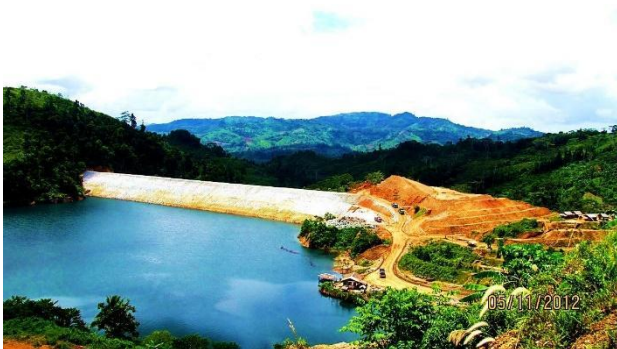
Canatuan Tailings Storage Facility – November 2012.
