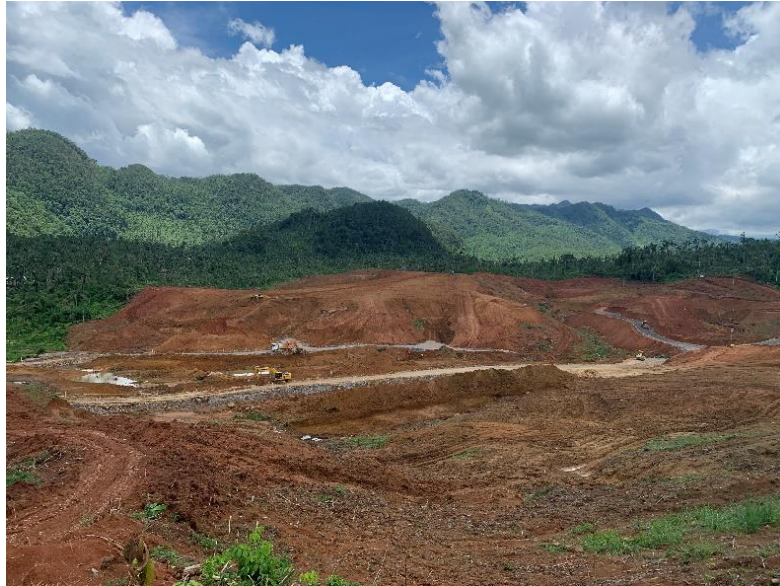
TSF6 construction at Siana Gold Mine on May 18, 2022.
