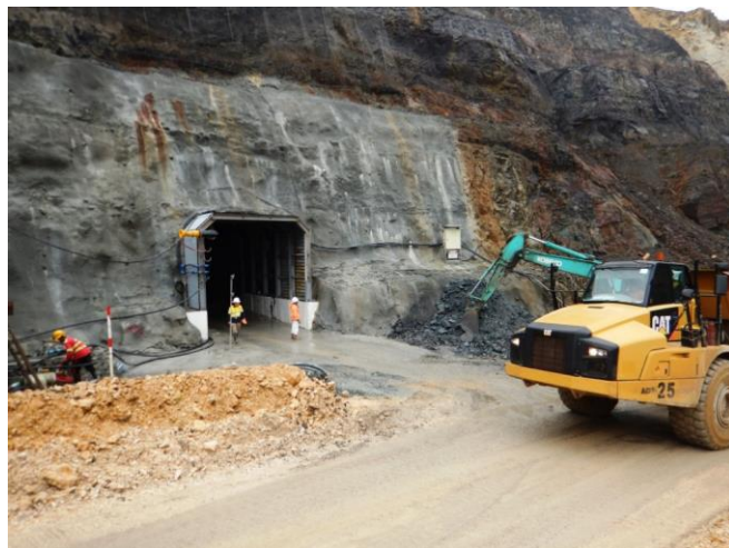
Construction of main access portal at the Siana Underground Mine. Source: Red 5 Limited March 2017 Quarterly Activities Report, dated April 28, 2017.
