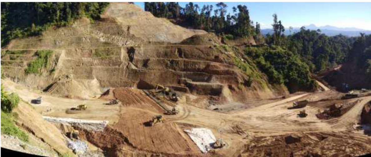
View of the TSF on November 23, 2020.
