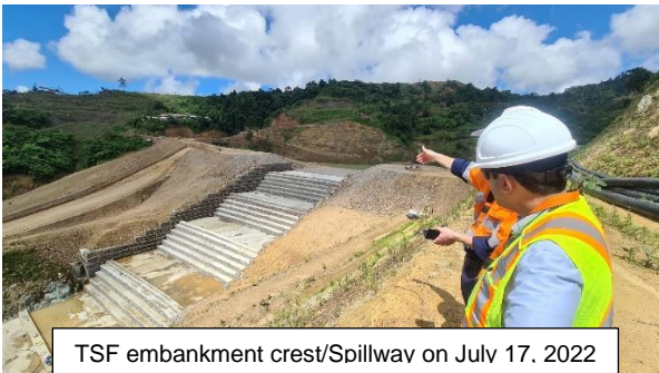
Gabion spillway step/drop/sidewall on July 17, 2022
