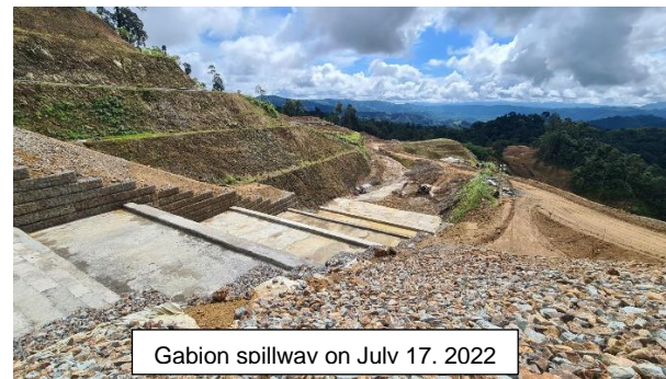
Gabion spillway step/drop/sidewall on July 17, 2022
