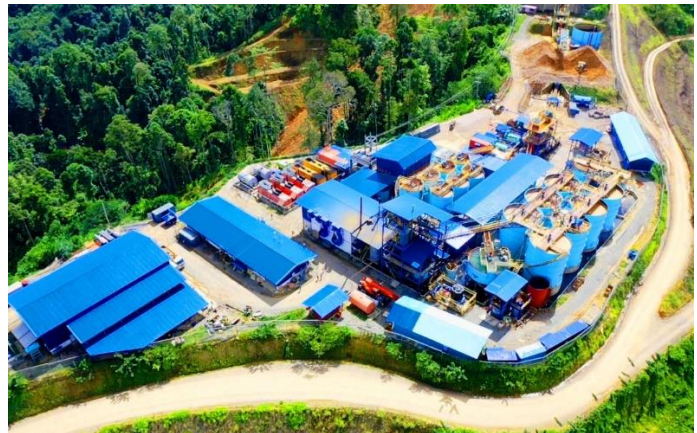
Aerial view of Mill Plant Site of the Balabag Gold Project on September 30, 2021.
