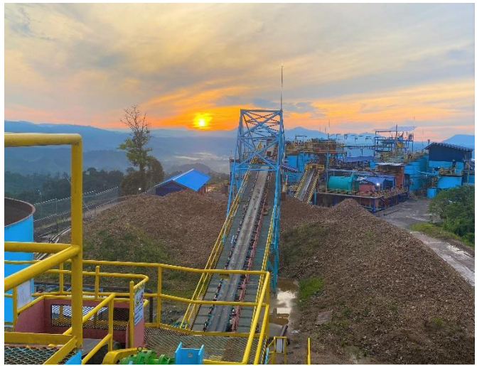
Views of the Process Plant on September 22, 2021.
