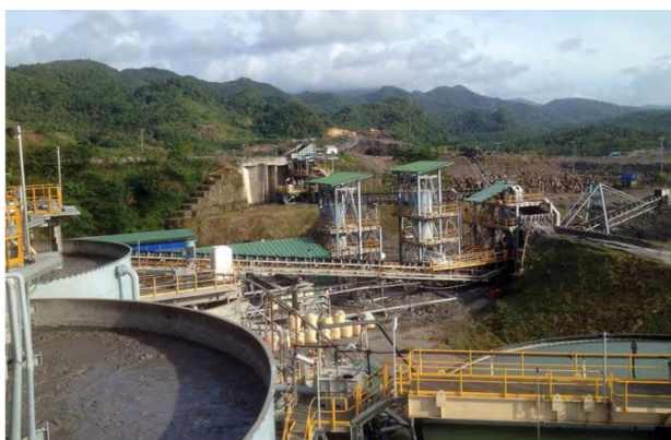
View of the Siana processing plant with the thickener and CIL tank in foreground.
