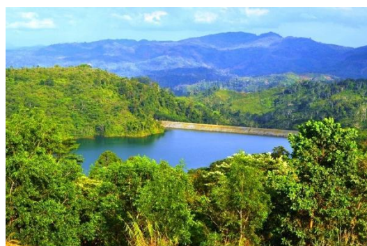
Canatuan Tailings Storage Facility – June 2020
