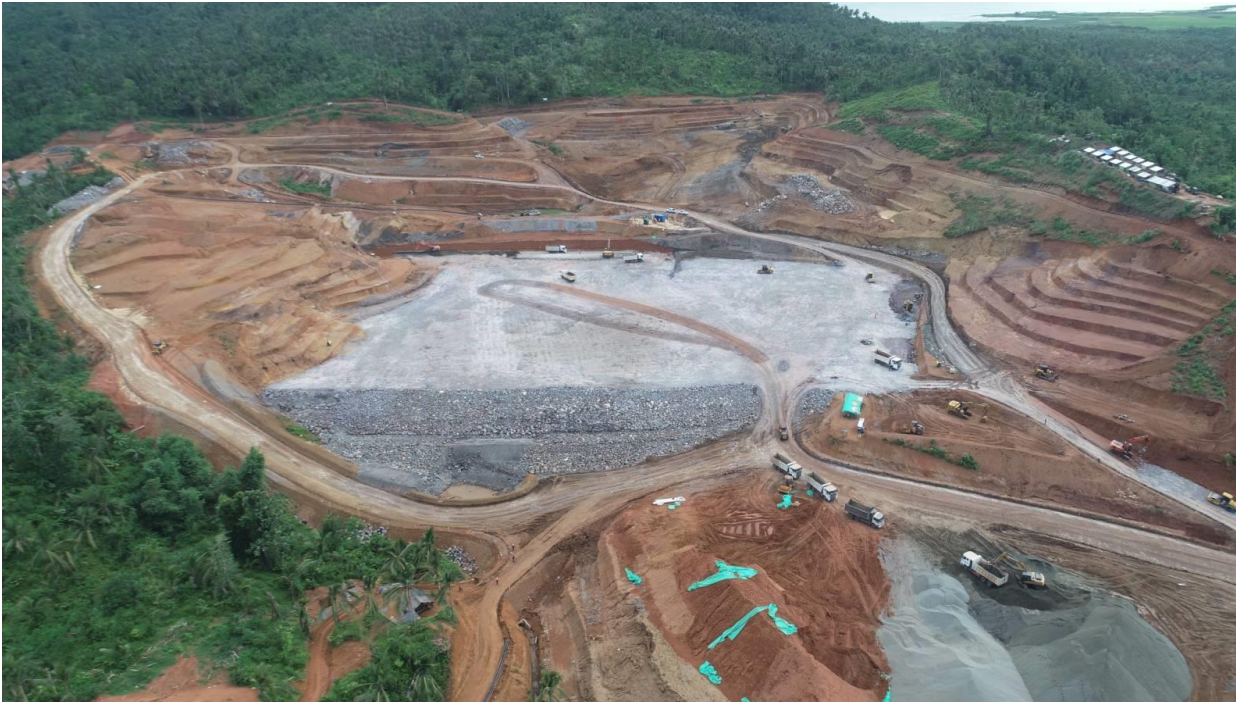
TSF6 embankment on October 3, 2022.
