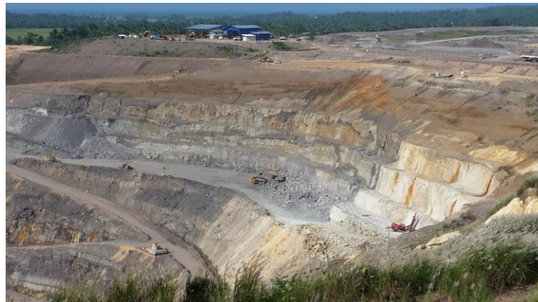
Mining west wall at Siana Gold Project.
