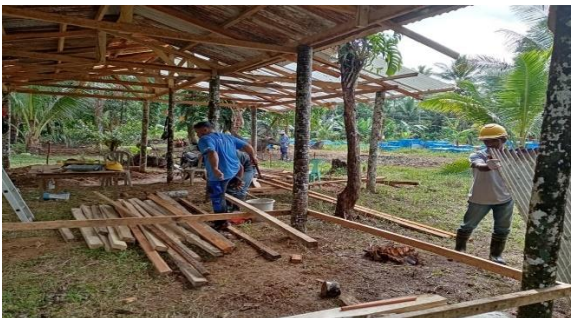
Construction of core house on October 25, 2022.
