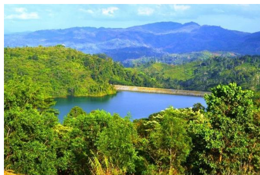
Canatuan Tailings Storage Facility – June 2021
