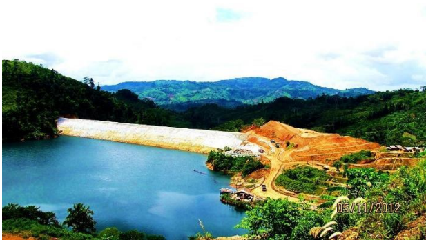
Canatuan Tailings Storage Facility – November 2012.
