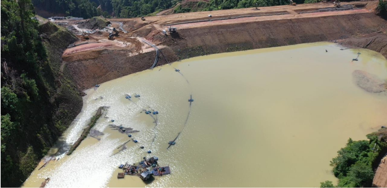
Installation of Pump #6 at the TSF on April 5, 2022.
