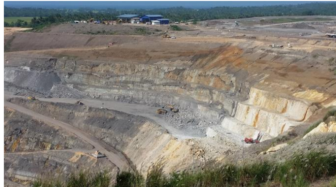
Mining west wall at Siana Gold Project.
