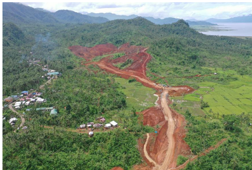
TSF6 construction at Siana Gold Mine on March 29, 2022.
