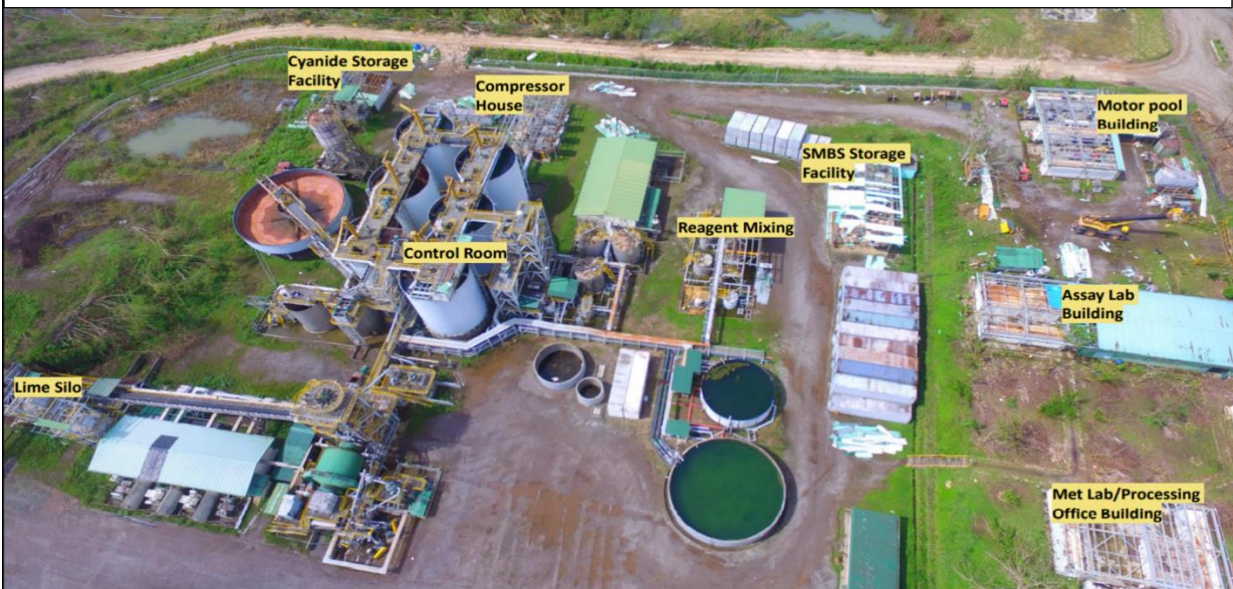
Aerial view of the Siana Gold Processing Plant on February 7, 2022.
