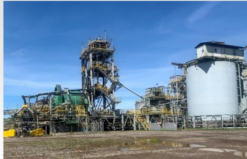
Photos: Views of the Siana Gold Processing Plant on May 18, 2022.
