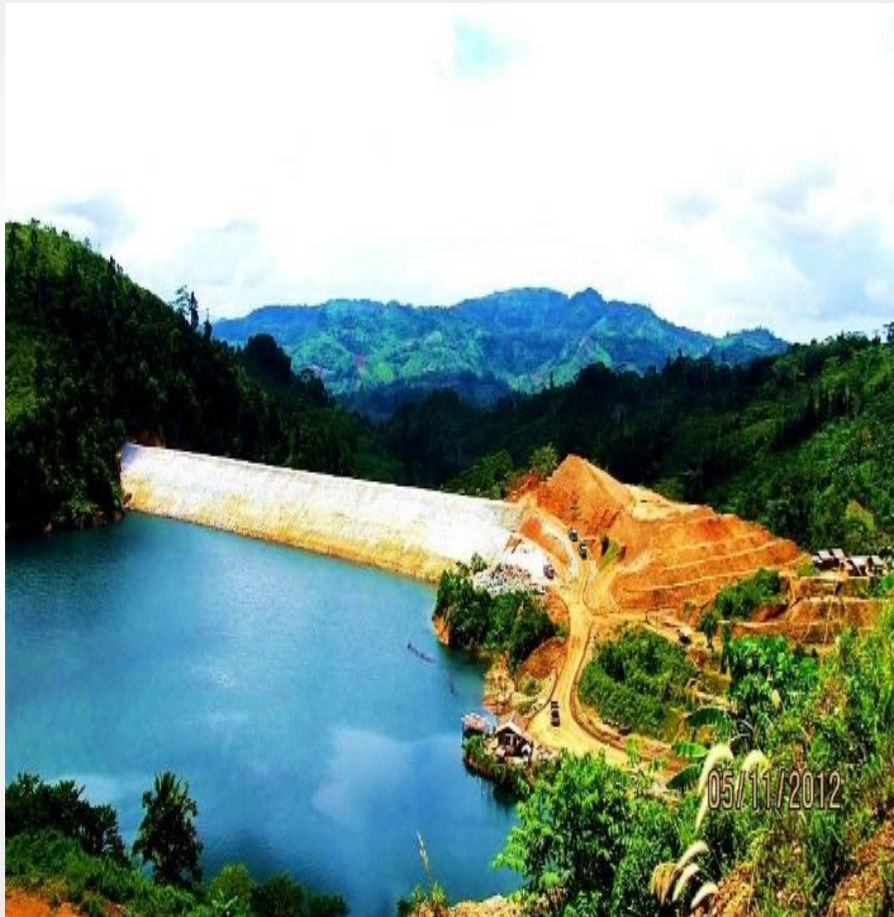
Canatuan Sulphide Dam – November 2012.
