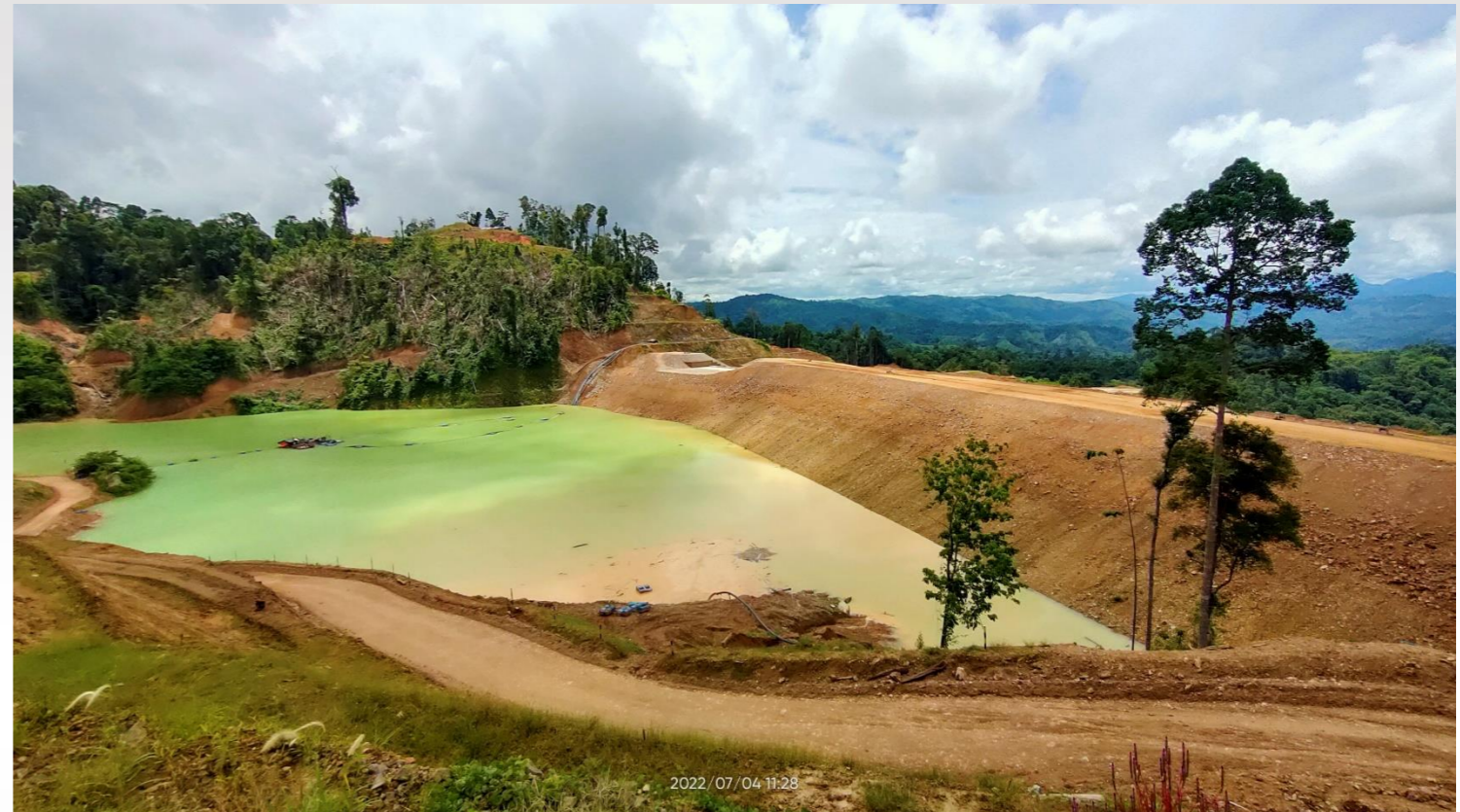
View of TSF impoundment on July 5, 2022.
