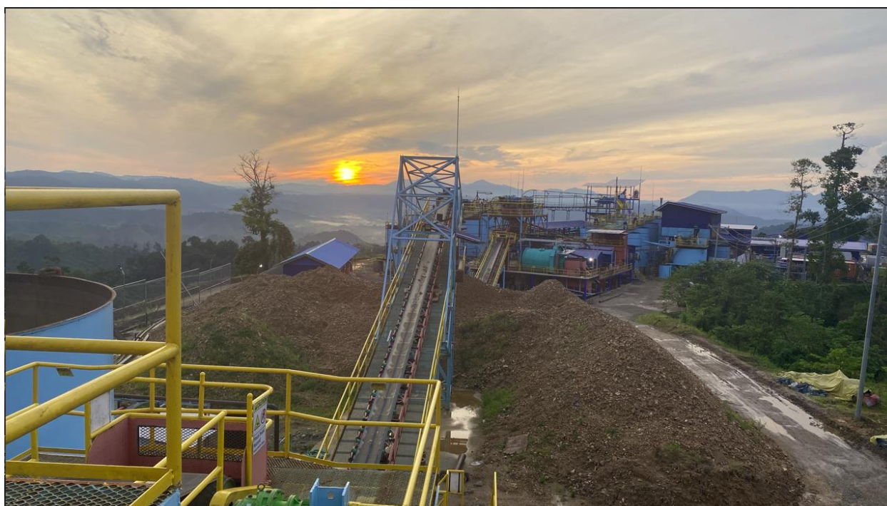
Balabag Gold & Silver Project process plant (June 23, 2024)
