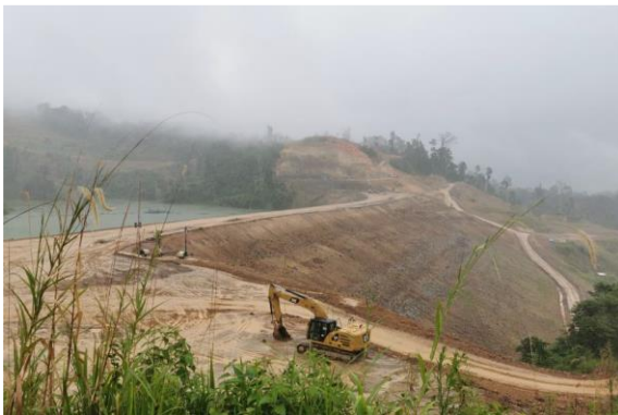
Balabag TSF construction: Ongoing placement of Zone 3A material at Stage 3B and spillway excavation on May 20, 2023.
