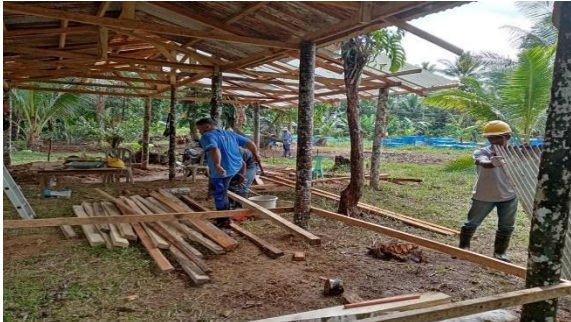
Construction of core house on October 25, 2022.
