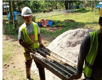
Core house activities at Mabilo – May 15, 2023
