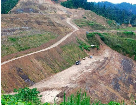
Balabag TSF construction: Stage 3B embankment placement. Photo: July 2023.
