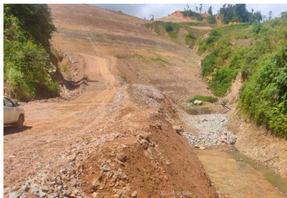
Balabag Stage 4 Valley Drain Photo: November 2023
