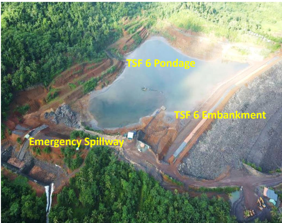
TSF-6, where the emergency spillway has been completed.
