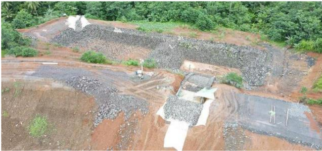
Emergency spillway construction.
