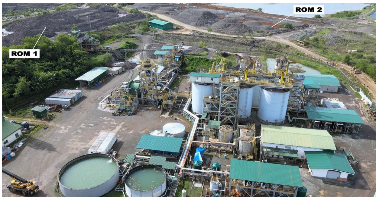
Siana Gold Processing Plant, April 5, 2023.
