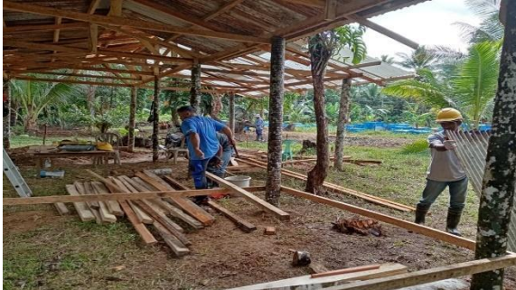
Construction of core house on October 25, 2022.
