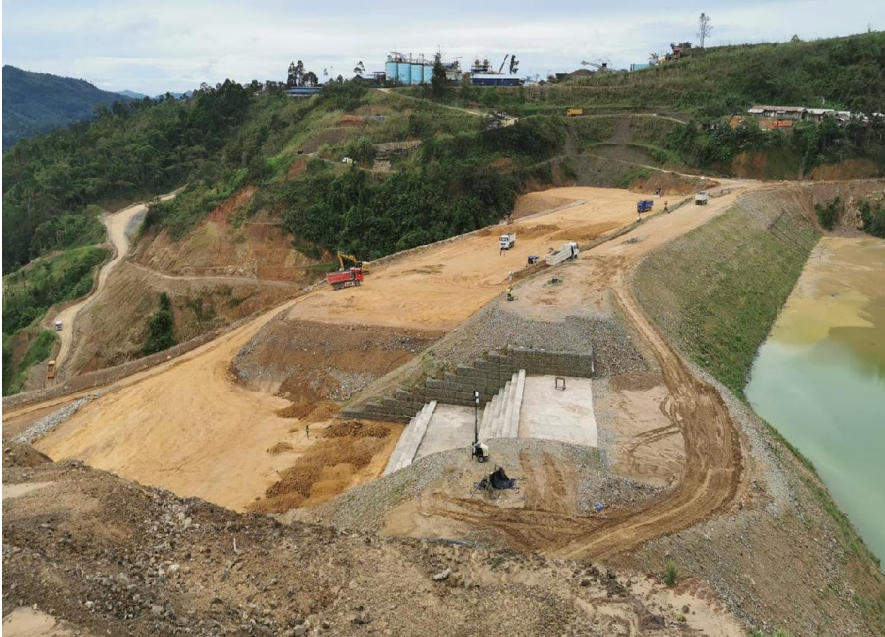
Spillway Stage 2 on January 12, 2023.
