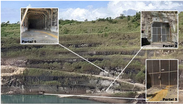
Current underground portals at Siana, April 2023, including Main Access, Exhaust Way and Return/Escape Way.
