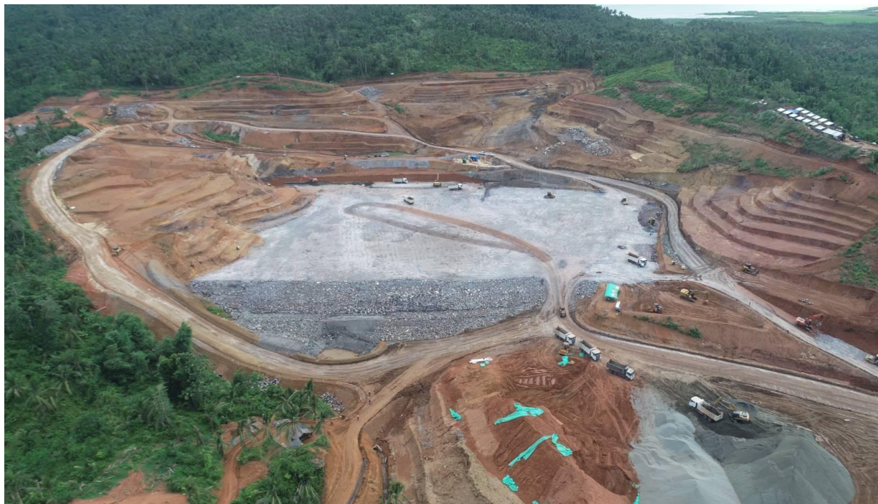
TSF6 embankment on October 3, 2022.
