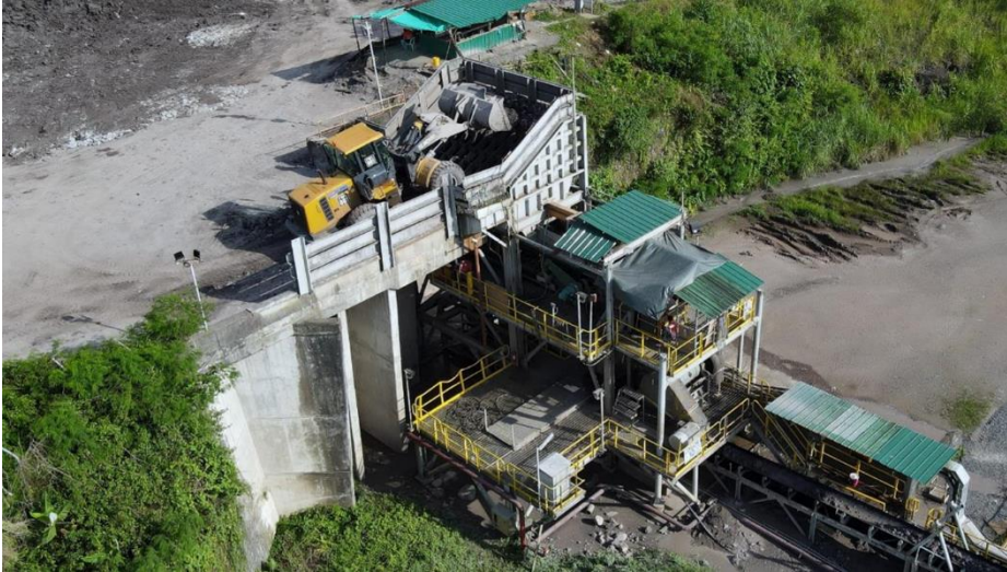
Siana Gold Crushing Circuit, April 5, 2023.
