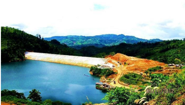
Canatuan Tailings Storage Facility – November 2012.
