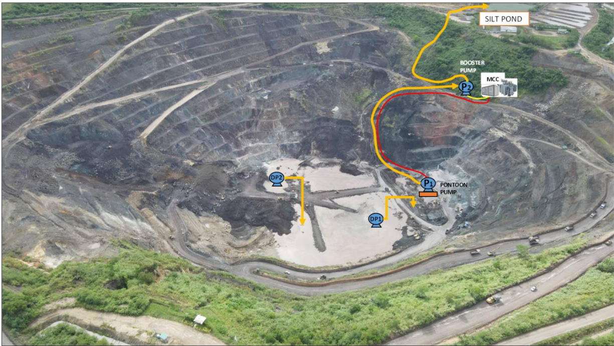
View of Siana open-pit mine and pit bottom recommended pump set-up - April 16, 2024
