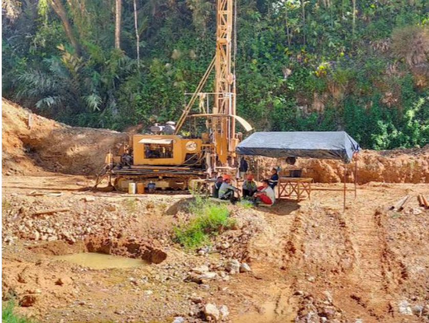
Ongoing geotechnical drilling. Balabag site – March 2024.
