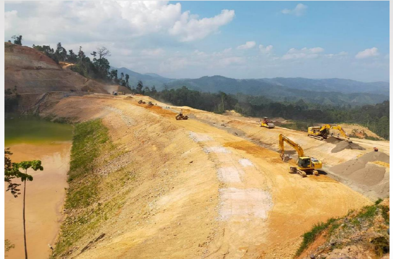
Balabag Tailings Storage Facility Zone 3A placement works on April 13, 2023.
