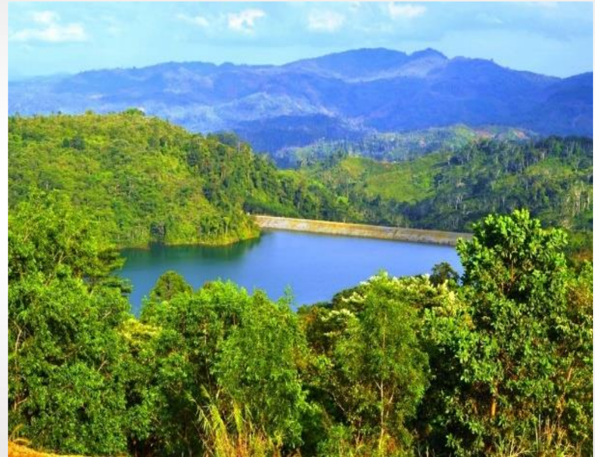
Canatuan Sulfide Dam – June 2020
