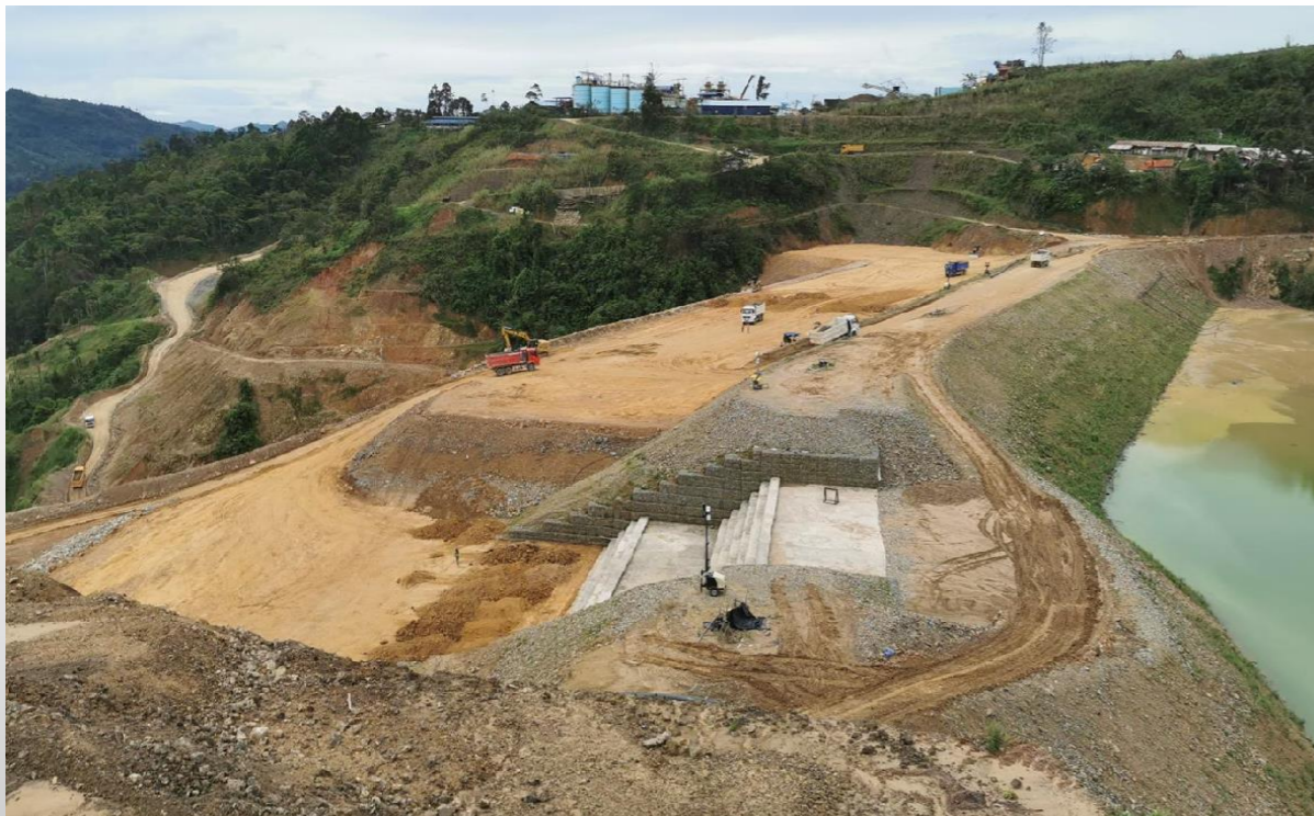
Spillway Stage 2 – January 2023.
