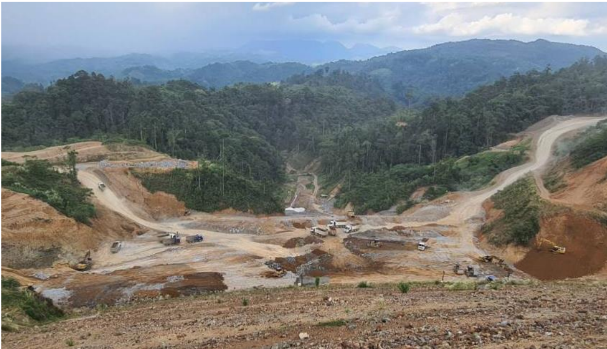
Stage 4 Downstream/Valley Drain: Embankment Activity – April 25, 2024
