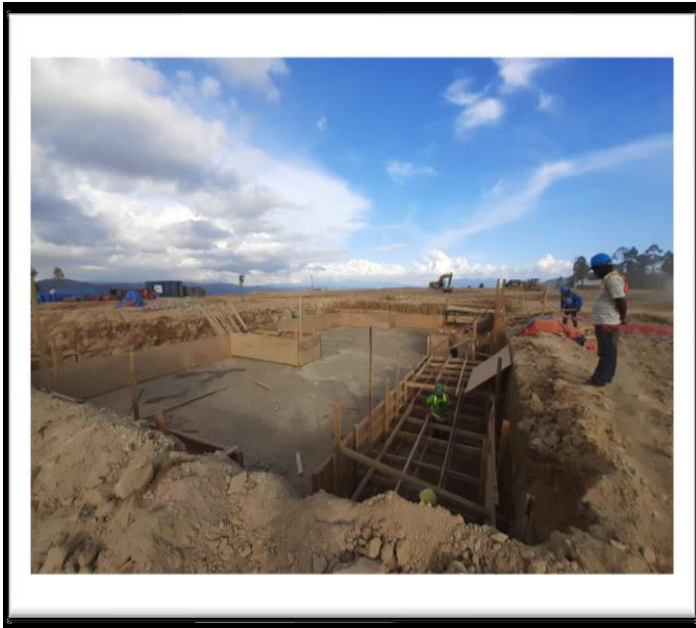
Installation of Forms Grinding-Foundation
