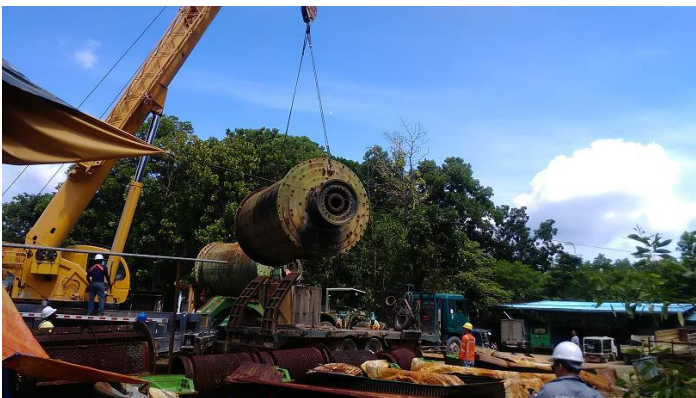
Installation of Forms Grinding-Foundation
