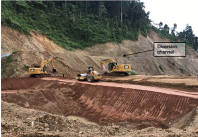
Upstream wall of the cofferdam.
