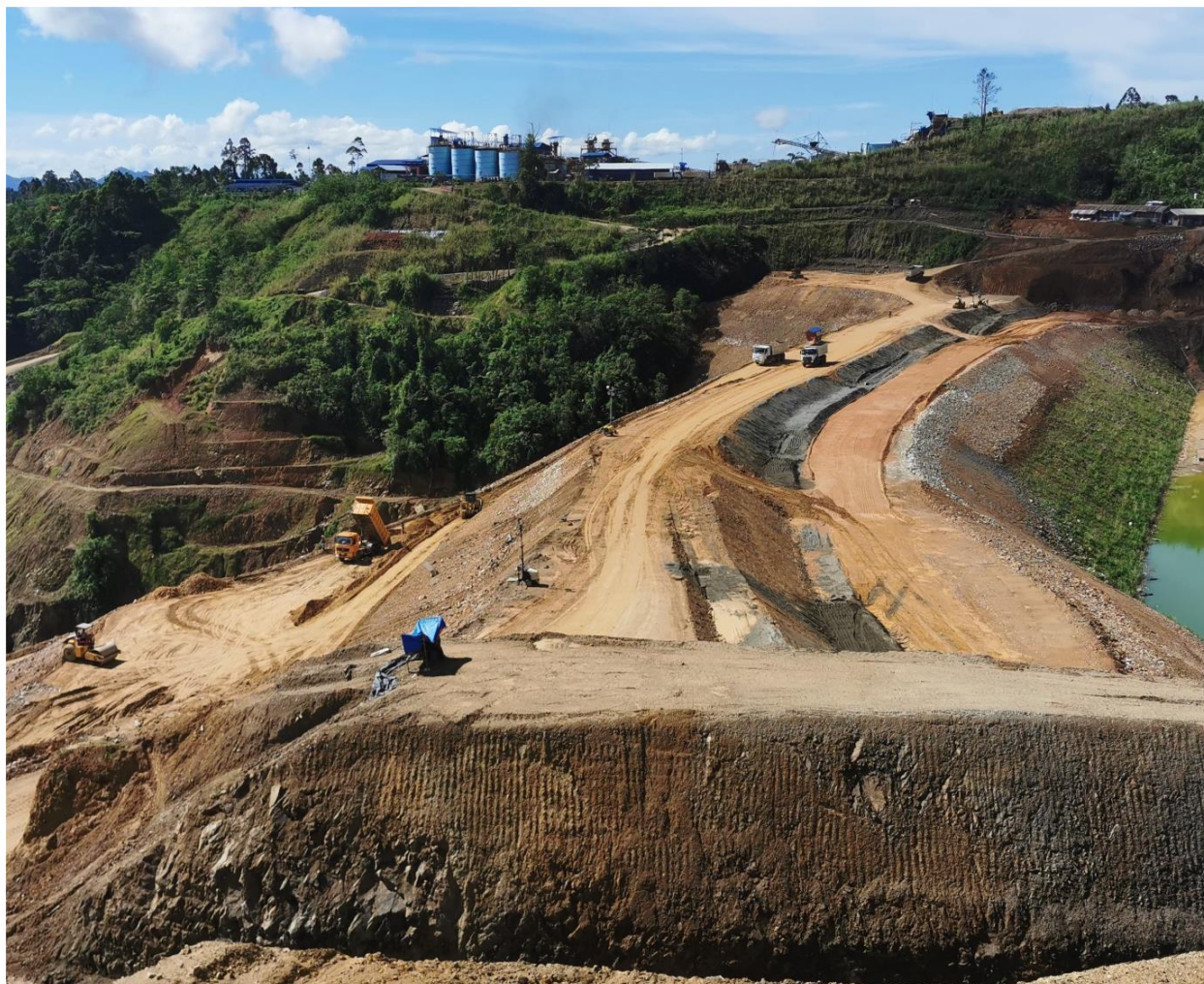
TSF embankment stage 3A progress as of March 25, 2023
