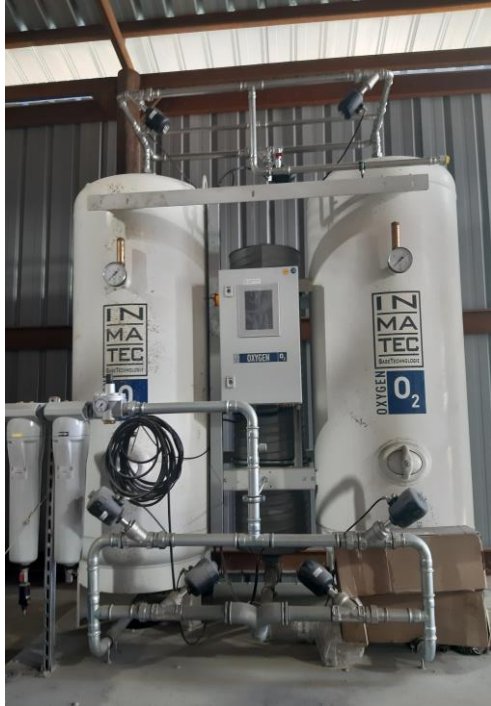
Installation of the oxygen generator in the leaching area of the Balabag Process Plant to further increase the efficiency of the cyanidation process (April 20, 2023).
