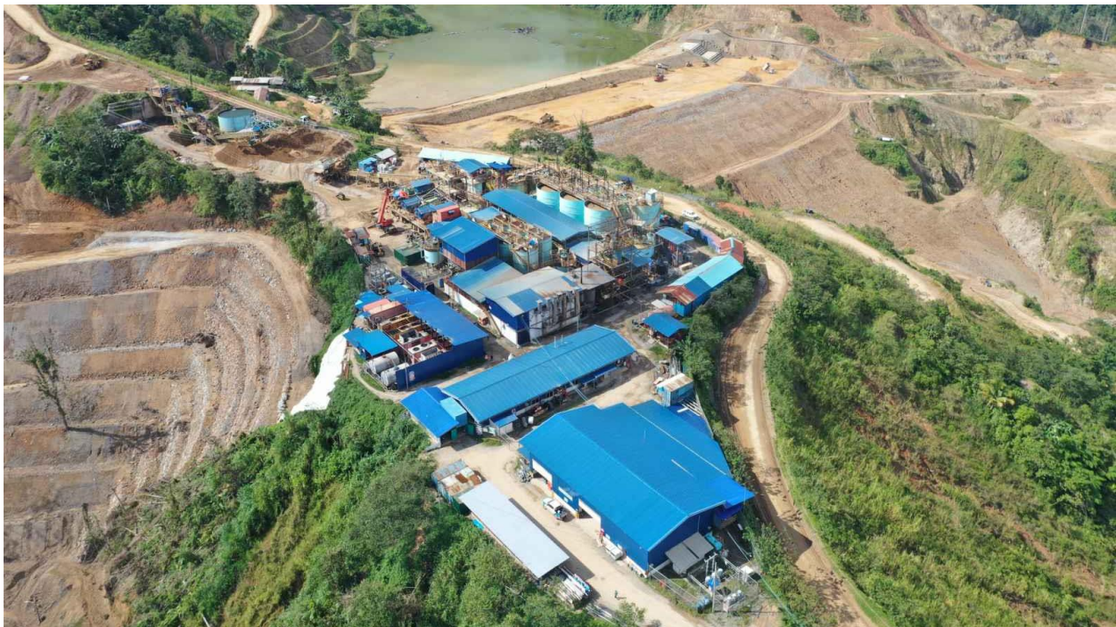
Balabag Processing Plant on February 23, 2023.
