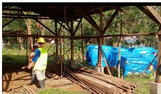
Construction of core house in October 2022.
