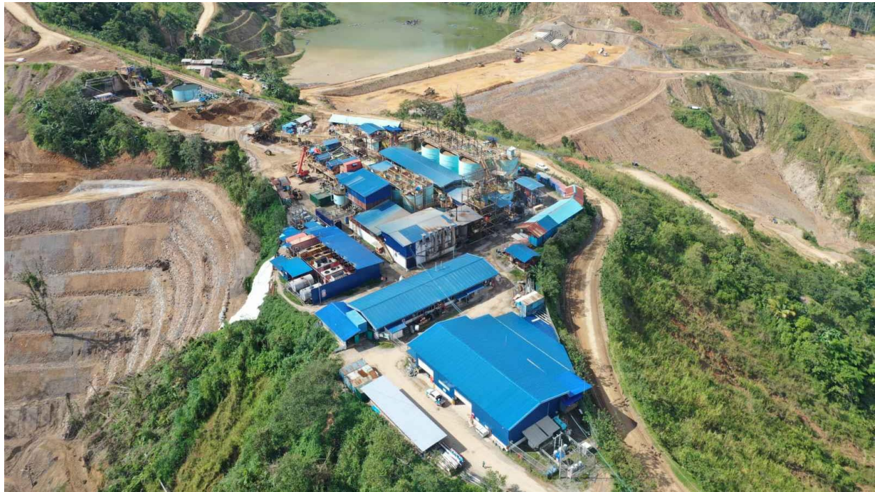
Balabag Processing Plant on February 23, 2023.
