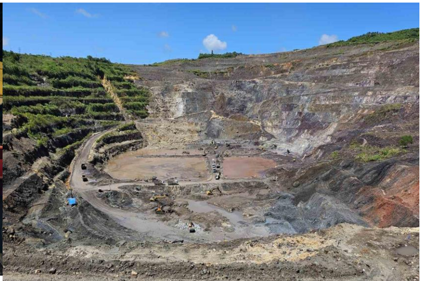
Siana pit development work March 23, 2024
