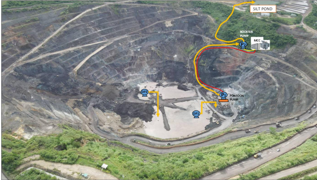
View of Siana open-pit mine and pit bottom recommended pump set-up - April 16, 2024
