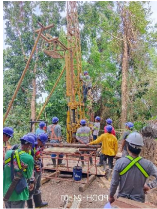
Drill rig setup
