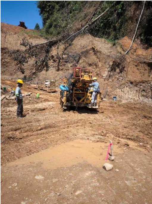
Exploration drilling April 23, 2026
