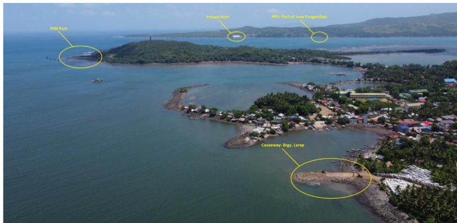
Aerial views of port/ causeway options being considered for the Mabilo Project (April 29, 2024)
