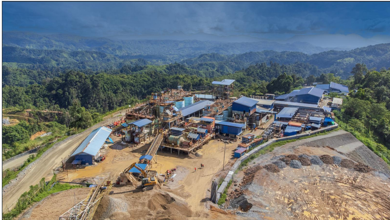
Balabag Gold Silver Project Process Plant (October 2025)
