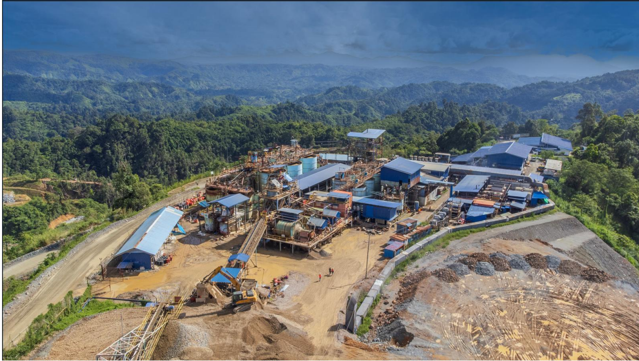
Balabag Gold Silver Project Process Plant (October 2025)
