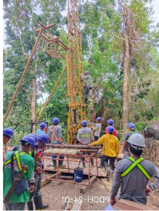
Drill rig setup
