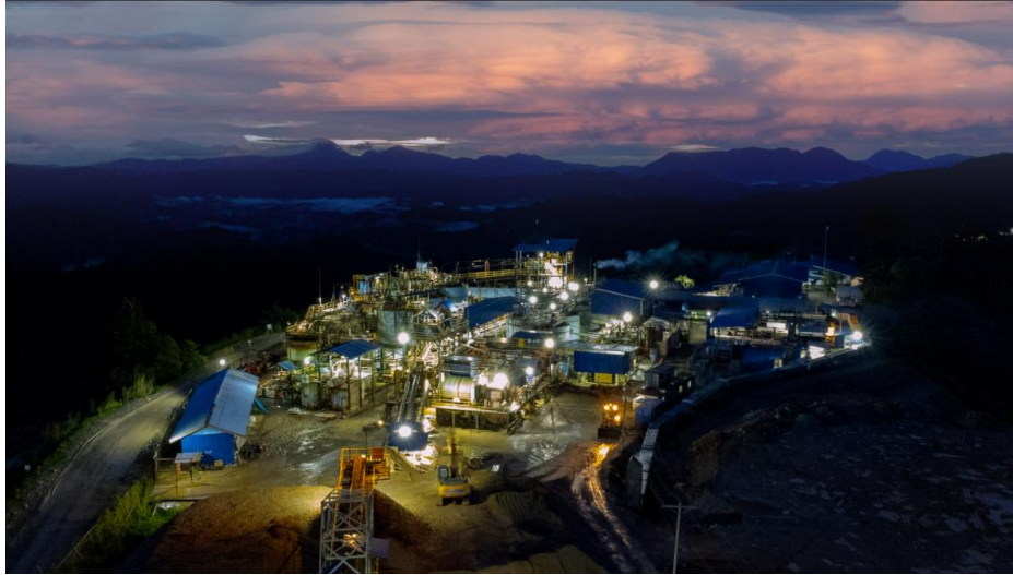
Balabag Gold Silver Project Process Plant (November 29, 2024)
